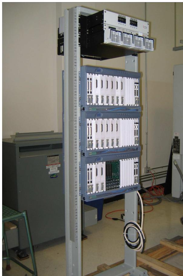
TDI's 4800 Watt Power System integrated with Zhone Technologies' MALC Broadband Loop Carrier systems.
